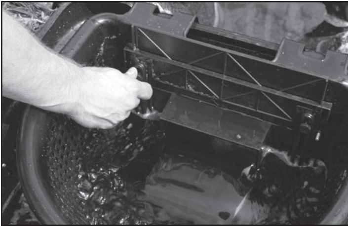
Fig. 32 Adjust the weir opening to the appropriate water level by loosening the thumbscrews.
