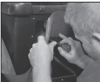
Fig. 13 Mark the outer perimeter of the skimmer opening on the liner; then mark a second box 1.5" inside mark. Cut out at inside mark.
